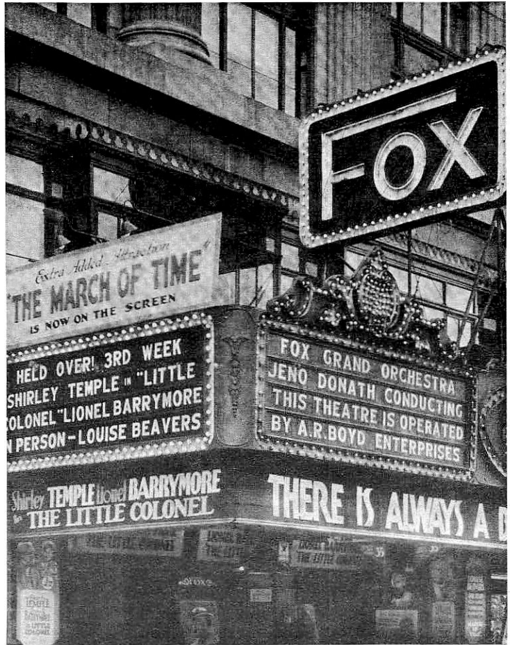
EMBELLISHED—Additions were made to the original Fox marquee, which can be seen in the exterior photos of the structure pictured at left and on preceding page. Not seen, but apparently added after the theatre had been in operation, were large verticle signs. —photo from Theatre Historical Society
